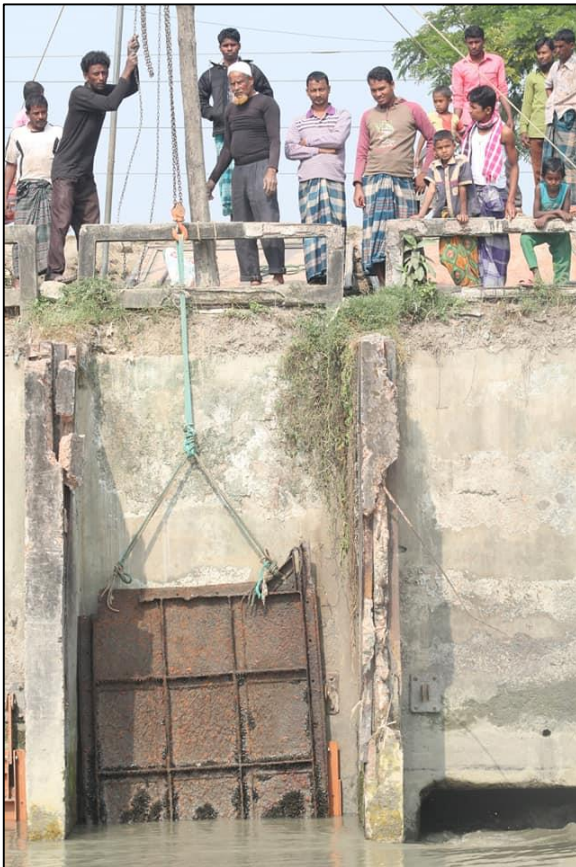
Figs: Replacement of damaged flap type water gates of a sluice-gate in Charfession
